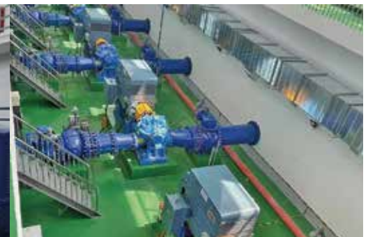
Anyang Western Water Transfer Project of South-North Water Transfer Project
