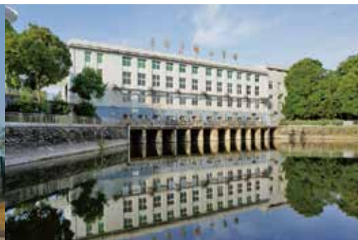
Mingshan Pump Station, Yiyang, Hunan
