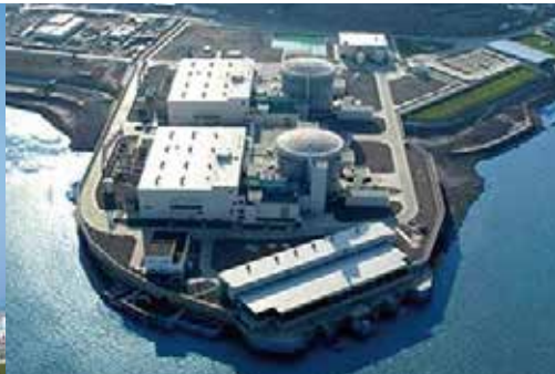
Fangchenggang Nuclear Power Station
