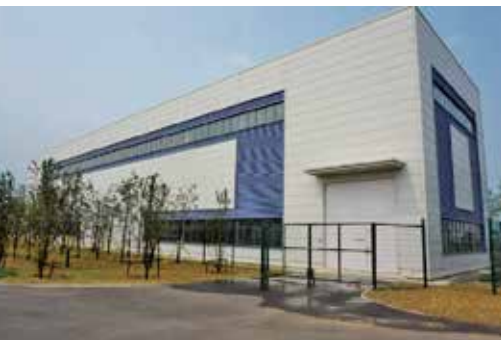
Tongzhou Water Plant Pump Station, Beijing
