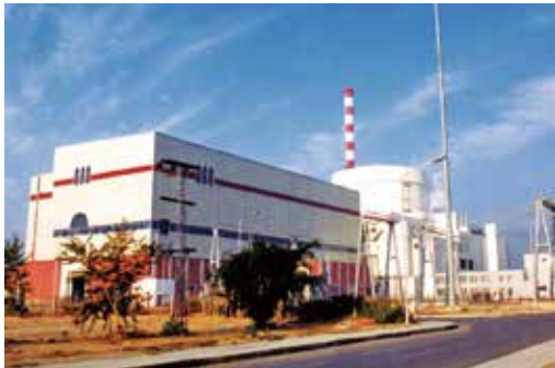
Chashima Nuclear Power Station in Pakistan, C3, C4 units
