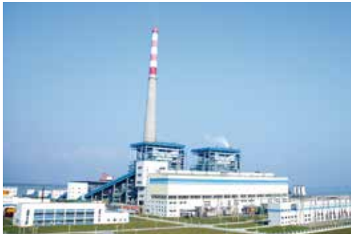
Beihai Power Plant
