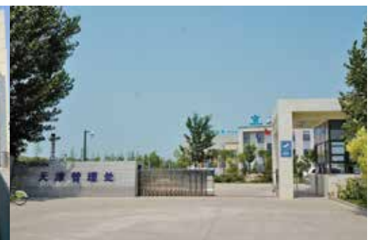
Caozhuang Pump Station of the South-North Water Transfer Project
