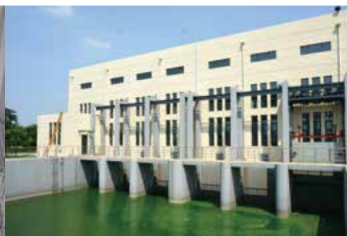
Tianjin Jinzhong River Pump Station
