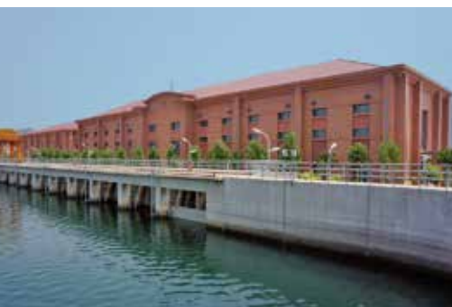
Tianjin Xi River Pump Station
